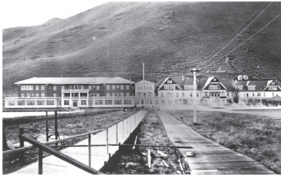
Hot Lake Sanitarium (southeast of La Grande) in its early days, ca. 1910s Building on left is the brick facility built in 1906; wooden buildings it replaced (right) were erected in the late 1800s and were destroyed by fire in 1934.
