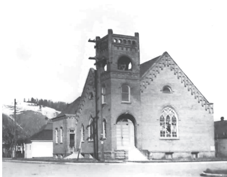
Baptist Church in La Grande, designed by Calvin Thornton, 1907 (now demolished)
